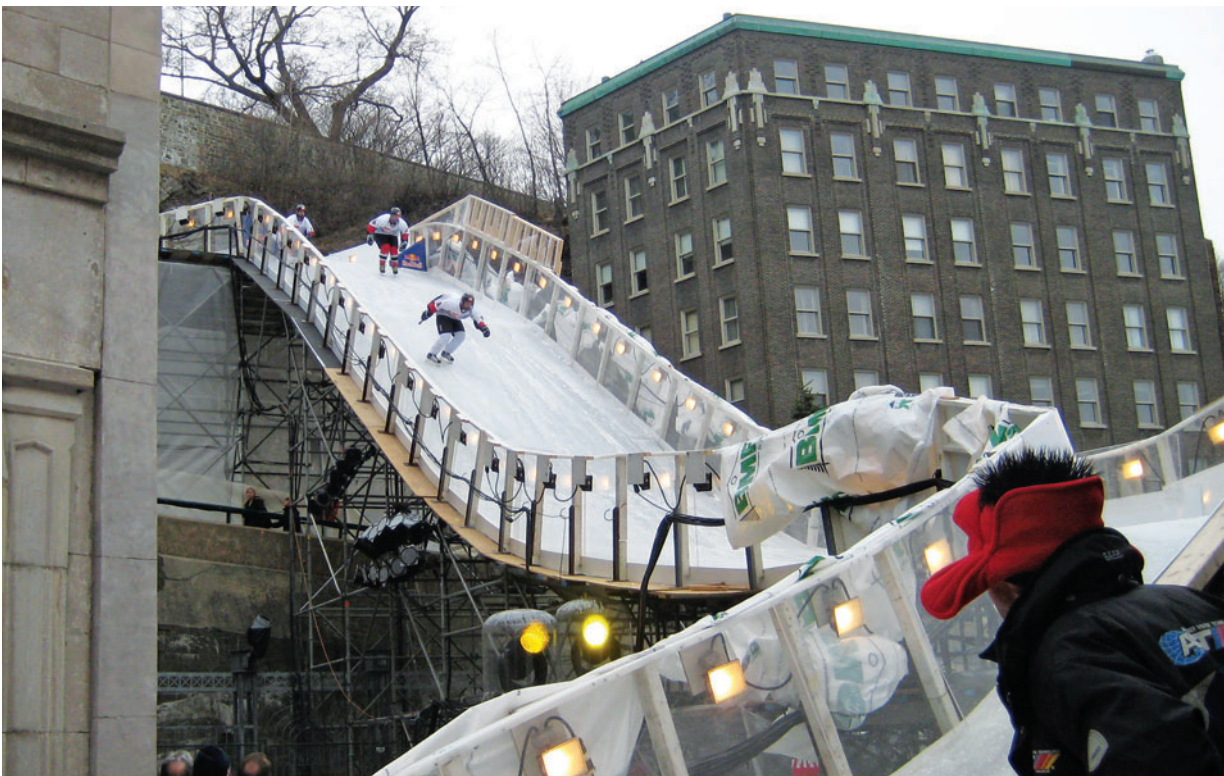
Big chillers and miles of piping kept the ice surface frozen for the Red Bull Crashed Ice competition in Quebec City.
